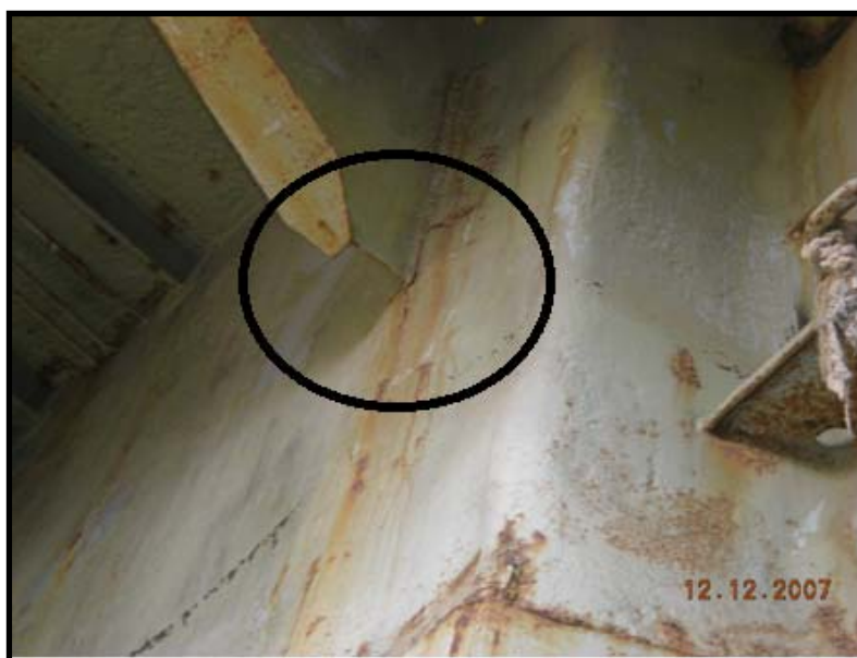
Fracture on transverse watertight hold bulkhead
