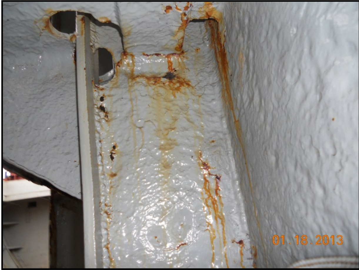
Figure 12. Holes on A Vertical Shell Plating Member Caused By Groove Corrosion
