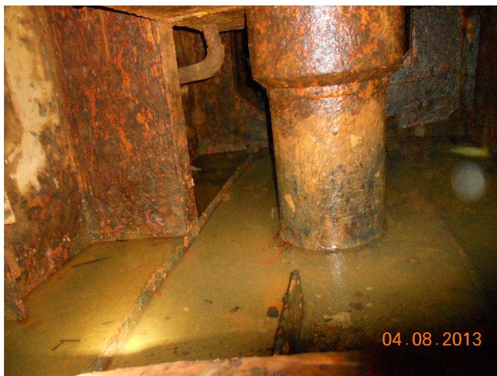
No safe access, and meaningful inspection not possible
