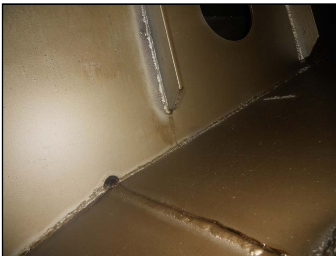
Fracture of web frame inside the topside tank
