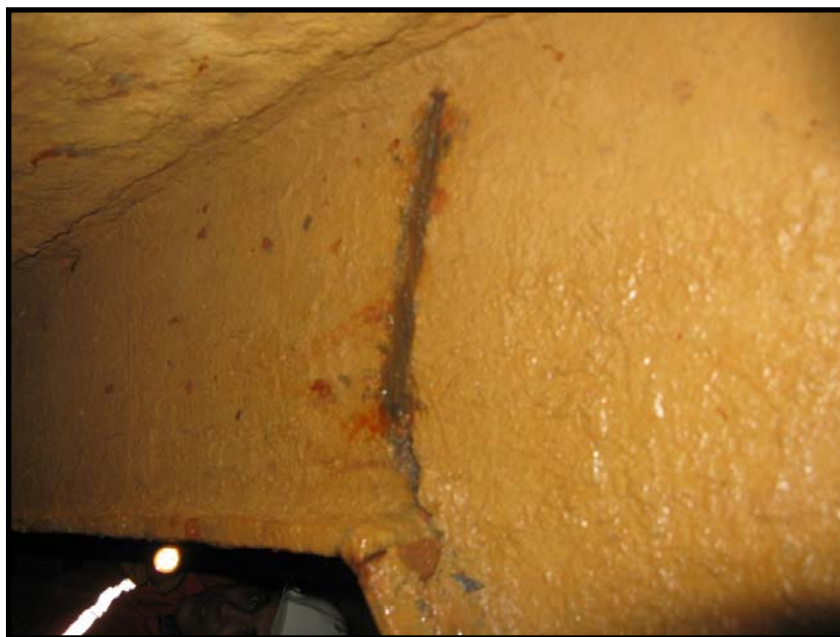
Fracture on shell frame inside a side tank
