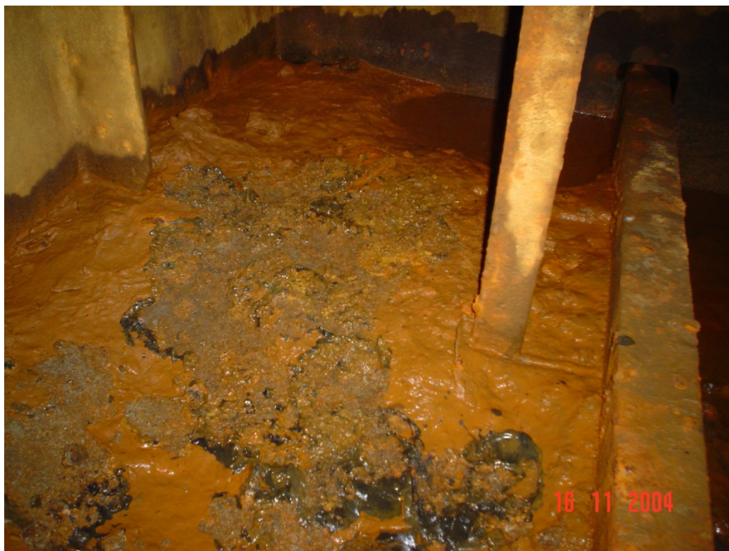
Large amount of sediments and water, bottom plating not visible
