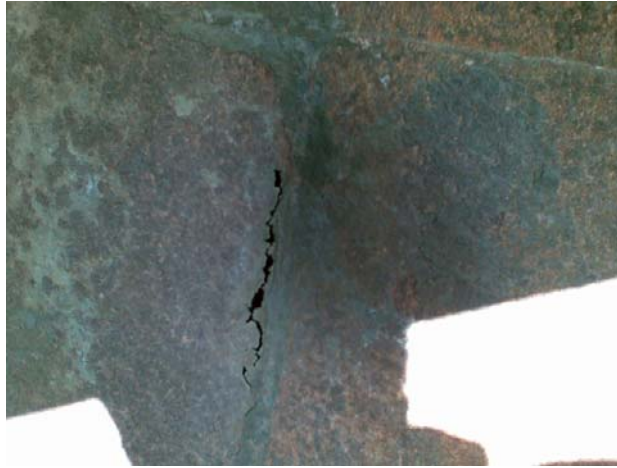
Fracture of weld joint on main deck
