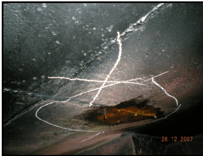
Fracture on bottom plating
