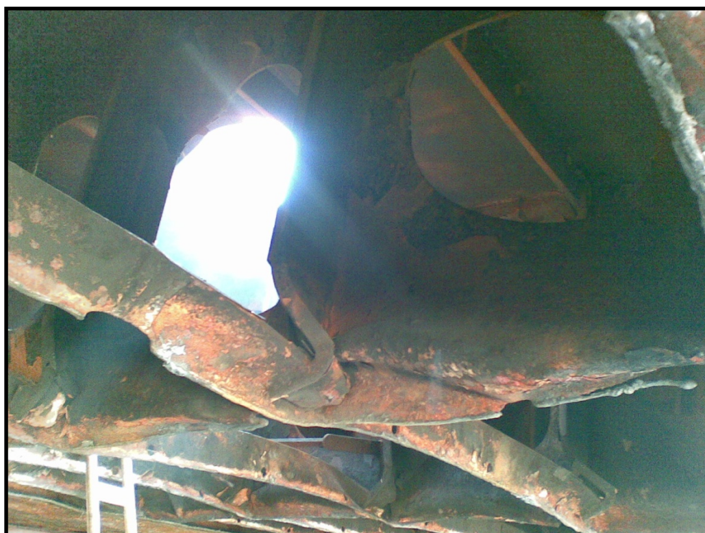
Multiple bays-deformed/tripped internals
