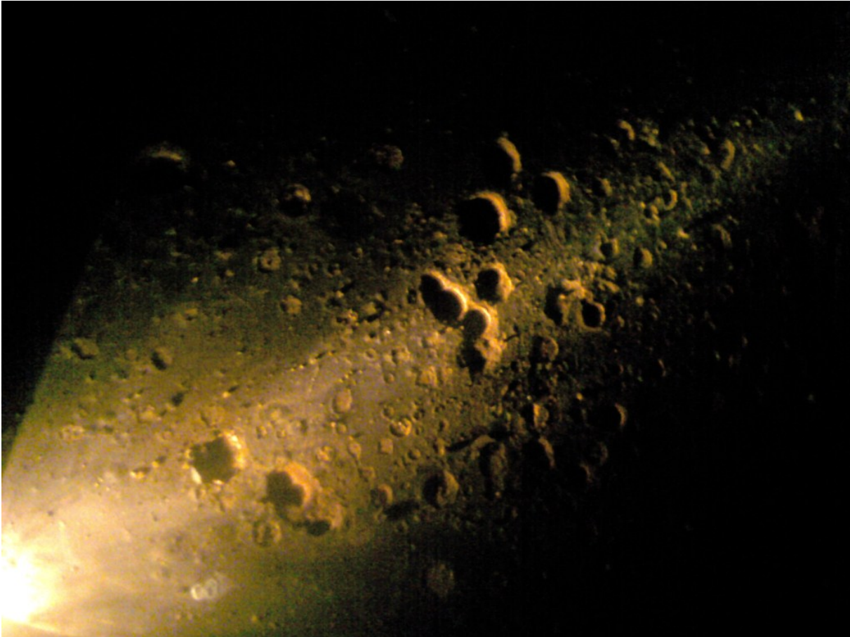
Figure 11. Pittings on Bottom Plating Inside A Ballast Tank
