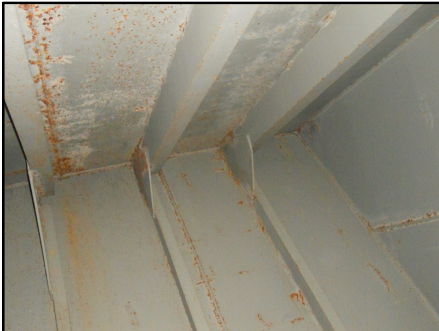
Newly coated,no major coating breakdown
